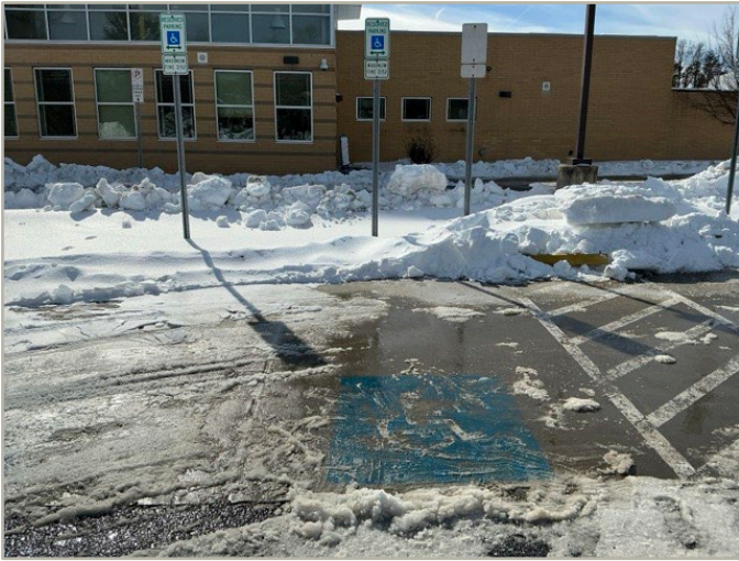
OVERVIEW OF ACCESSIBLE PARKING AREA
