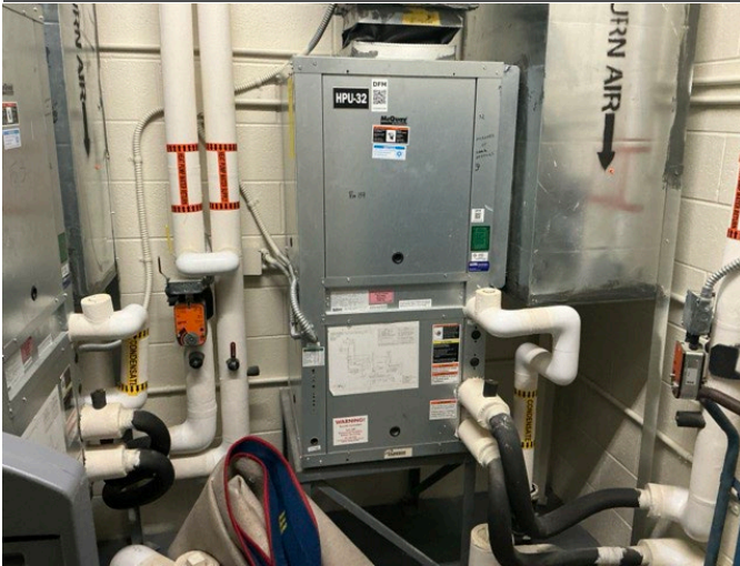
25 - WATER SOURCE HEAT PUMP
