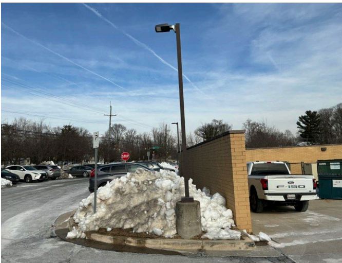
39 - PARKING LOT LIGHTING
